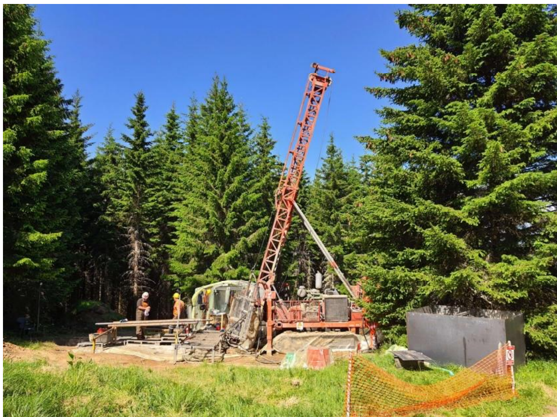
Figure 2: Drill Rig II - in operation
