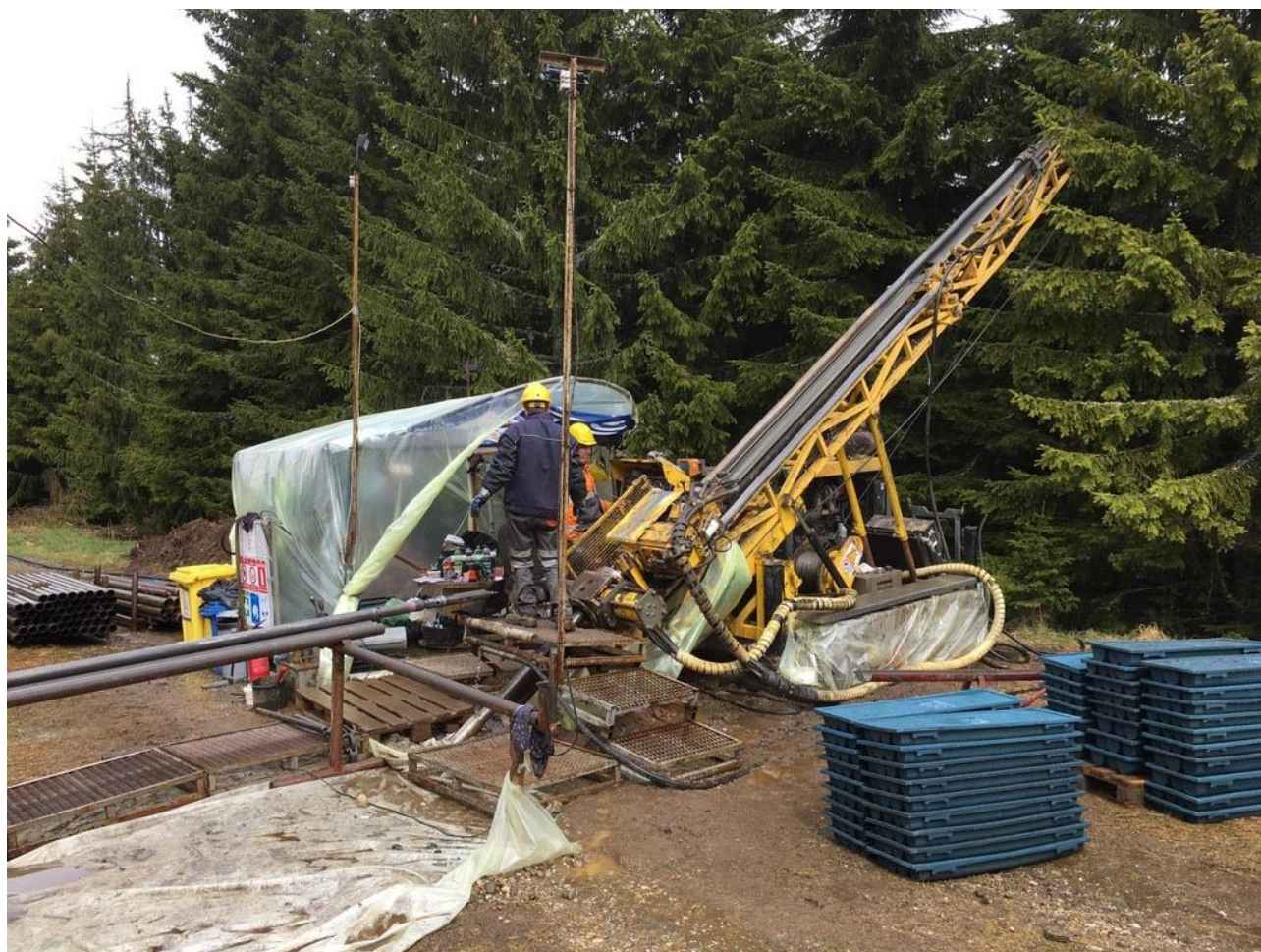
Figure 1: Drill Rig I - in operation
